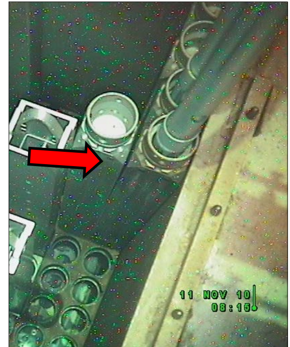
SAFARI-I Original Beryllium Reflector Elements Photo Courtesy of NECSA, South Africa
